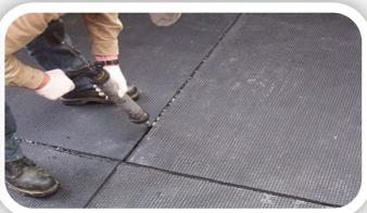
Quattro's range of high density mats can be bonded to new and existing floors using our Matbond urethane resin. The resin expands as It cures to take a hold of the grooves and joints In the mats from underneath. Once the mats are in place the joints between the mats are cut out using a heated rubber groover. The cut strip is then removed to leave a clean open groove.
