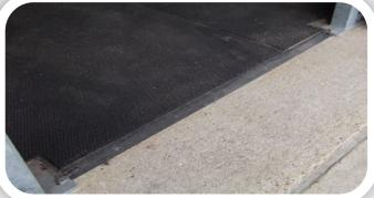
The joints are then sealed using our Q/Flex Gun applied flexible urethane resin as well as the perimeter of the area. Any residual sealant left on the surface of the mats will be removed with use.
