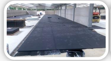
Quattro's range of high density mats can be bonded to new and existing floors using our Matbond urethane resin. The resin expands as It cures to take a hold of the grooves and joints In the mats from underneath.
