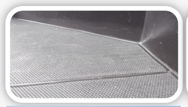
The joints are then sealed using our Q/Flex Gun applied flexible urethane resin as well as the perimeter of the area. Any residual sealant left on the surface of the mats will be removed with use.
