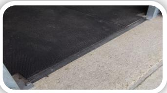
Heavy duty plastic doorway strips are fitted in to doorways or along drains to protect the edge of the mats if no thresholds in place.
