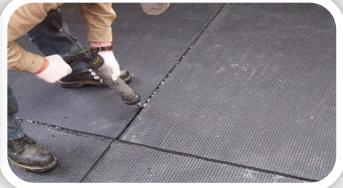
Once the mats are in place the joints between the mats are cut out using a heated rubber groover. The cut strip is then removed to leave a clean open groove.
