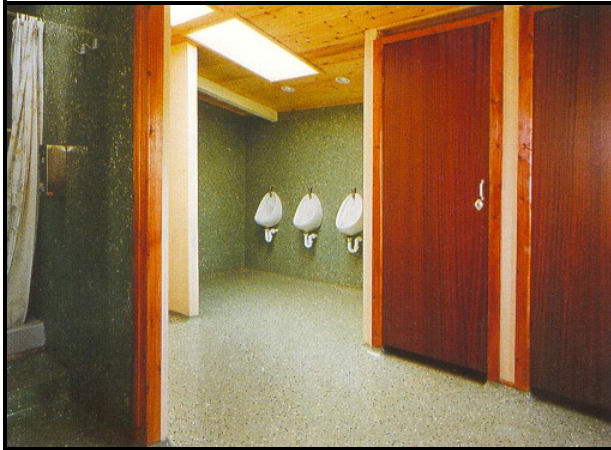
SEMI-FLAKE FLOOR AND WALLS SHOWING MOST OF BASE COLOUR
