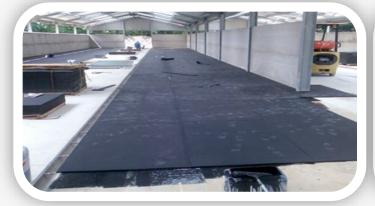
Quattro's range of high density mats can be bonded to new and existing floors using our Superflex Membrane The specially developed rubber adhesive achieves a strong bond to the rubber mats and subbase.
