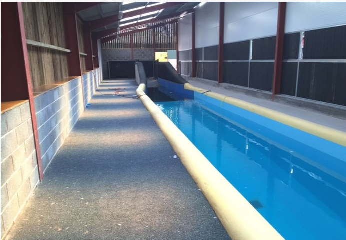
Flexscreed to Pool Surround & Q/Tyle Gloss to Pool Walls
