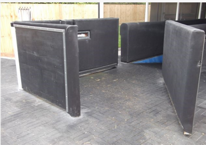
Brick Effect Tiles to Pool Surround and Equiflex Wall Padding
