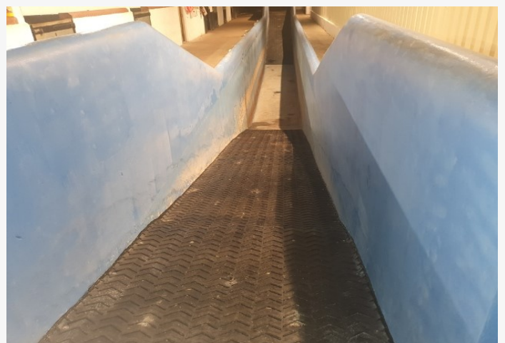
Chevron Matting to Ramp
