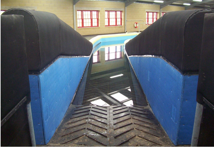
Equiflex Padding & Eva Mats to Walls. Chevron Matting to Ramp
