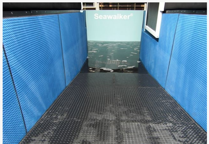
Grip Top Tiles to Ramp and Eva Mats to Walls of Seawalker
